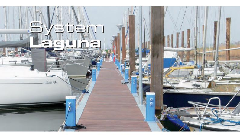
The Laguna system is a modular aluminum pontoon solution. These modern pontoons are very durable and practically maintenance free. They are suitable for sheltered locations where there is a high risk of corrosion.
